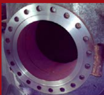
Resurfacing raised face flanges
